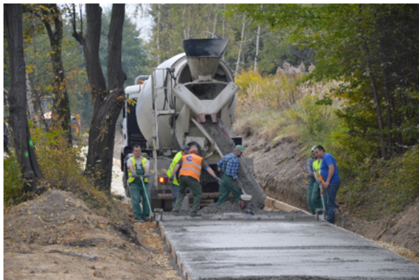
Figure 6. Local government road construction with the use of a vibrating strip
