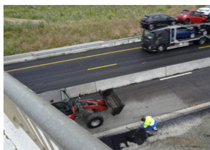
Figure 7. Temporary solutions - workzone protection
