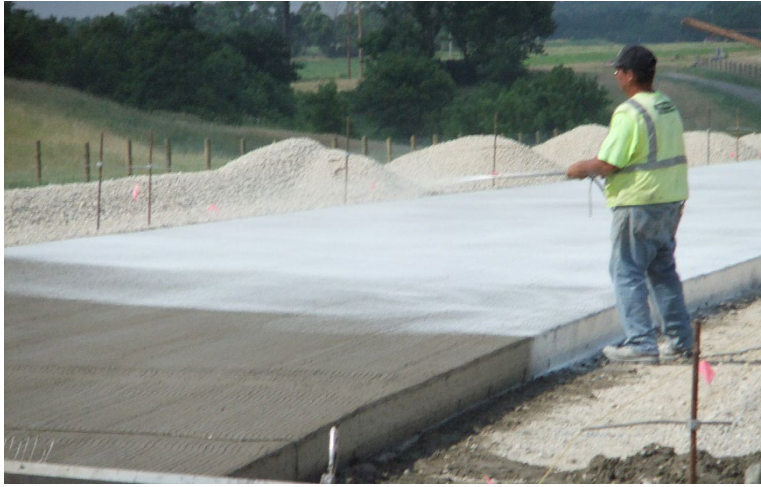
Figure 3. Protection of the concrete with a curing compound.
