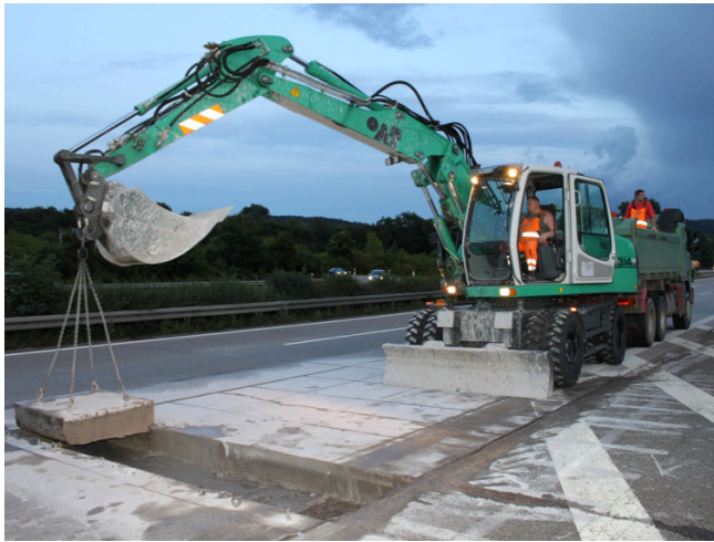
Image 4. Vibration-free lifting and removal of the damaged slab
