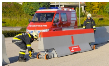
Figure 5. Special systems - a removable barrier section
