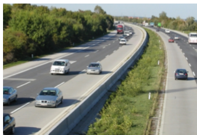
Figure 2. A concrete central reserve or median barrier
