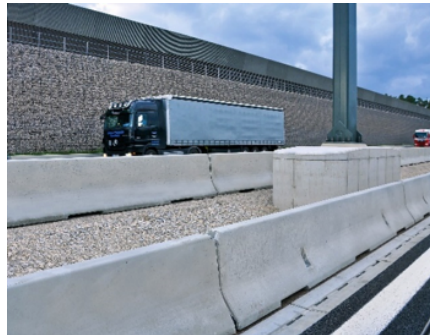
Figure 13. Anchored, semi-rigid system
