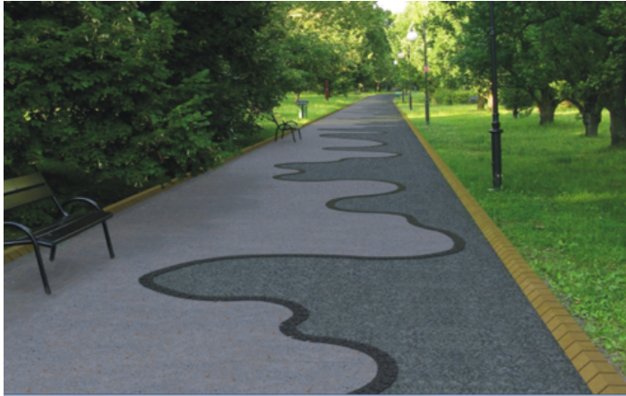
Figure 10. Decorative concrete pavement – Warsaw, a path in the park
