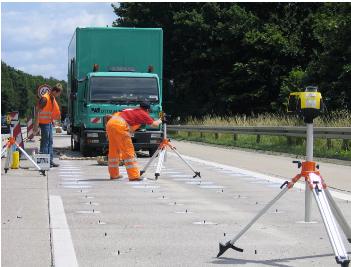
Image 3. Position monitoring with laser measuring technology and step gauge
