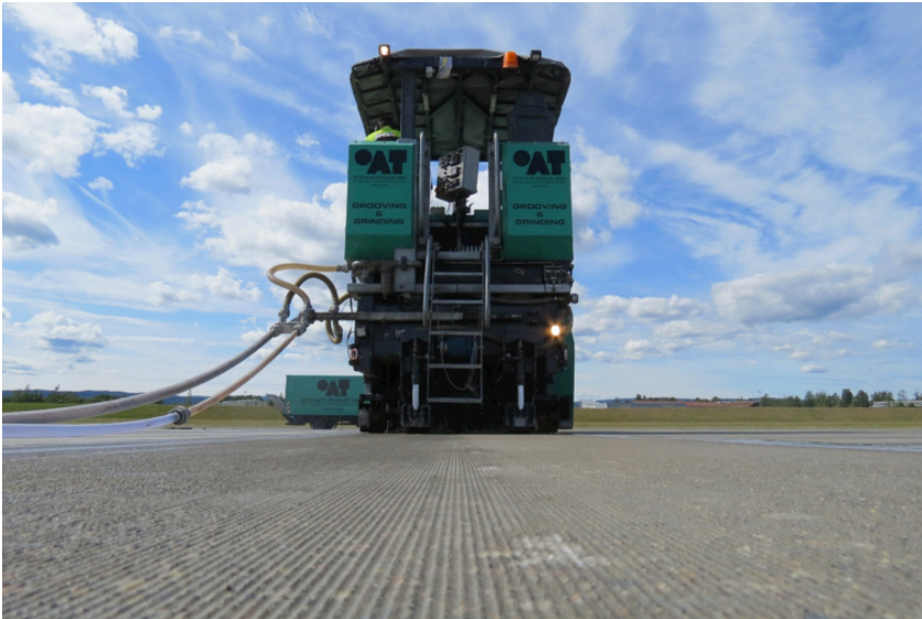
Image 2. Surface structure with fine grinding grooves
