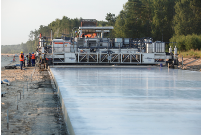
Figure 5. Motorway A1 in construction in the vicinity of Łódź (2015)
