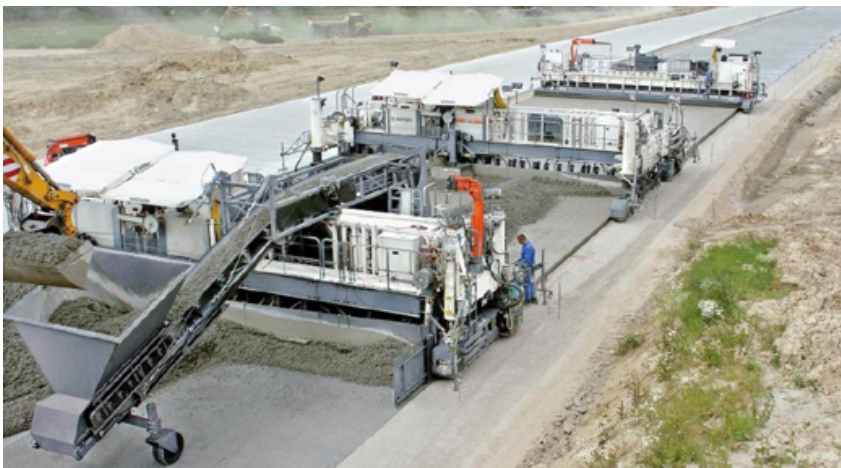
Figure 6. Two layer paving with two machines
