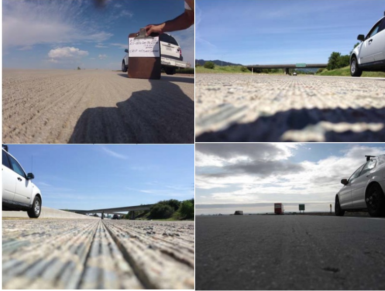
Figure 3. Examples of concrete pavement textures (a) longitudinal tining, (b) diamond ground (c) diamond-grooved, and (d) surface burlap-drag
