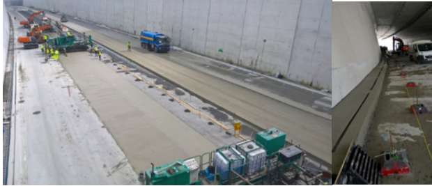
Figure 7. Construction of the two-layered concrete in the open trench and tunnel
