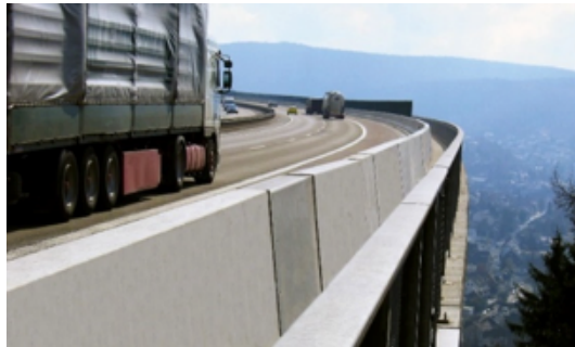
Figure 3. A concrete bridge parapet
