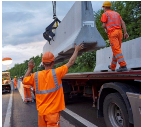
Figure 15. Installation of concrete barrier elements
