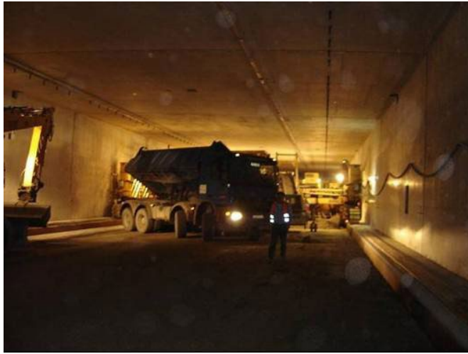
Figure 3. Side dump truck (1)
