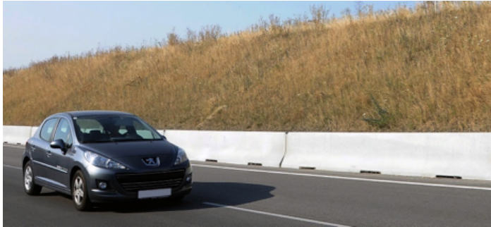
Figure 1. A concrete hard-shoulder barrier
