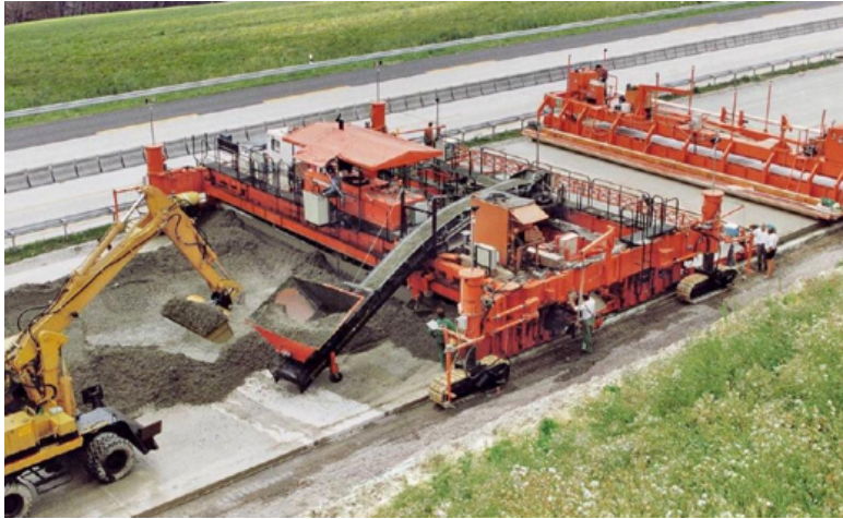
Figure 7. Two layer paving with one machine
