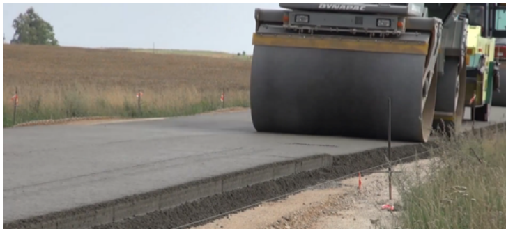
Figure 9. Construction of local government road using roller-compacted concrete technology
