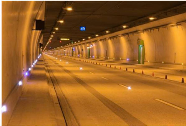
Figure 2. The Juan Carlos I Tunnel in Spain with a jointed slab concrete pavement (1)
