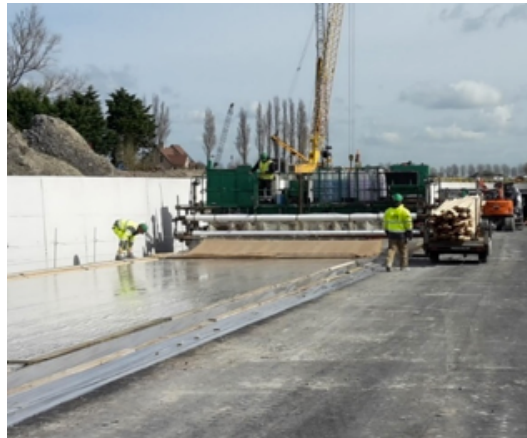
Figure 10. Placing and securing of the plastic sheet with wooden beams
