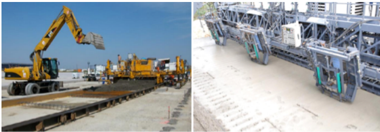
(a) Dowels and tie bars on baskets (b) Automatic dowel and tie bar inserter
