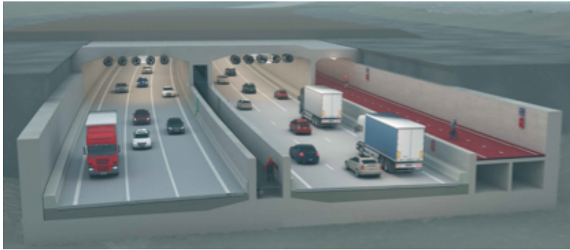
Figure 15. Tunnel under the river Scheldt, with CRCP as road pavement
