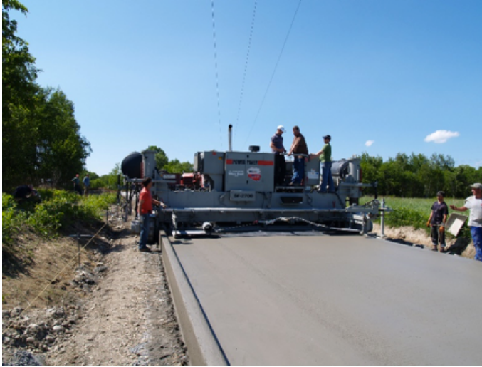
Figure 7. Construction of local government road using slip formwork and the paver
