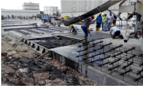
Figure 1. The Concrete Road Production
