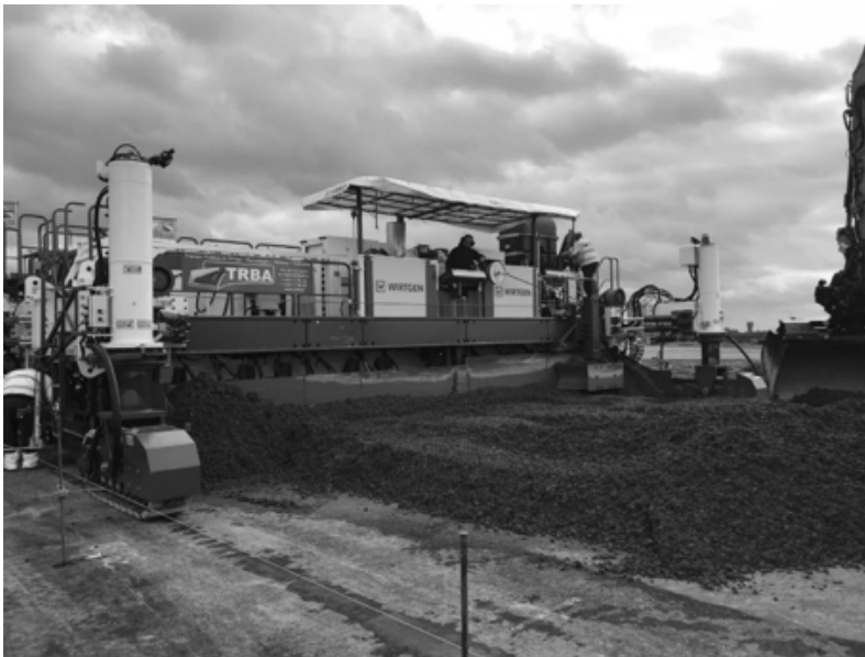
Figure 2. The SP 1500 on the A7/E42 construction site.
