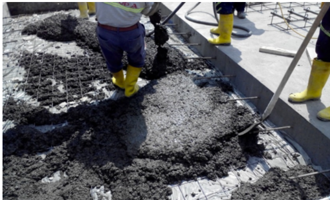
Figure 2. Application of the Concrete
