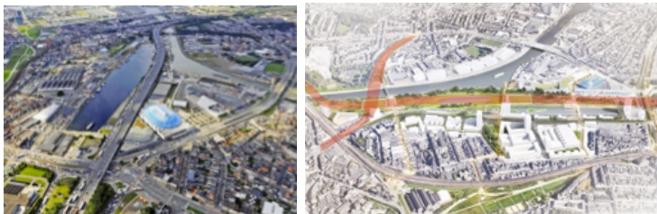
Figure 14. Rehabilitation of the area above the new tunnels of the Oosterweel link – before (left) and after (right)
